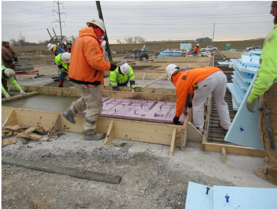
A crew works on tilt-up wall panels that will be installed at the new St. Louis Blues practice facility in Maryland Heights, Mo.
